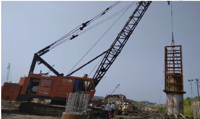
Dynamic Load Test in progress
